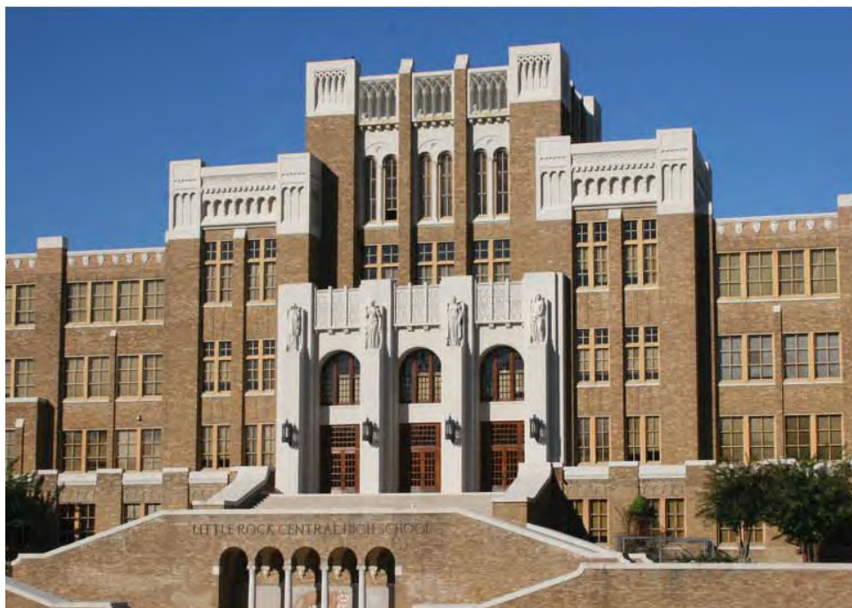
Figure 2-174b. These photographs show very little change to the facade of Central High School since the period of significance. However, two evergreen trees that flanked the main entrance are no longer extant. Source: John Milner Associates, Inc., 2007.
