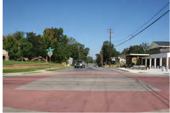
Figure 2-49. A scored and tinted concrete paving pattern has been recently installed at the intersection S. Park Street and Daisy Bates. Source: John Milner Associates, Inc., 2007.
