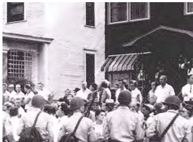
Figure 3-2. Metal awnings at 1501 S. Park Street. Source: Central High Museum, Inc., Coll B-12.I.65, ca. September 1957, National Park Service, Little Rock Central High School National Historic Site (detail).
