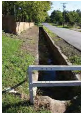
Figure 2-145. A drainage canal along Jones Street that begins at W. Sixteenth St. Source: John Milner Associates, Inc., 2007.
