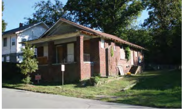
Figure 2-104. Boarded-up Craftsman bungalow on W. Sixteenth St. Source: John Milner Associates, Inc., 2007.
