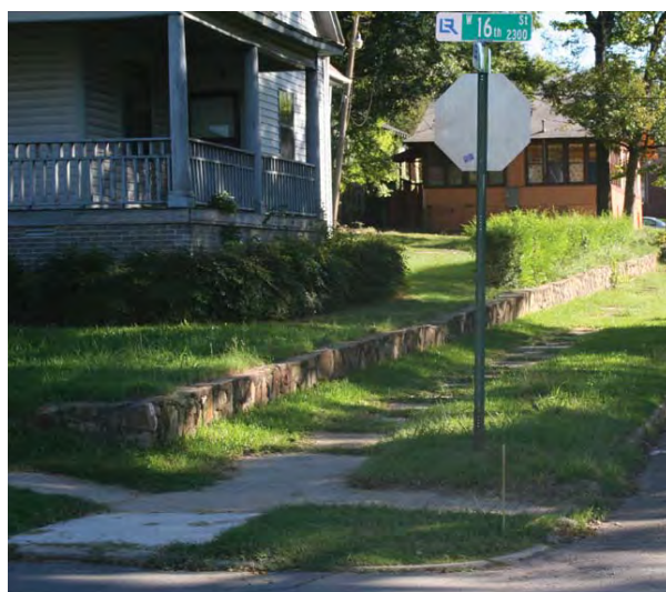
Figure 2-159. Raised lot supported by low retaining wall. Source: John Milner Associates, Inc., 2007.
