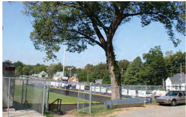
Figure 2-114. Chain link fence surrounds many areas within the school ground. Source: John Milner Associates, Inc., 2007.
