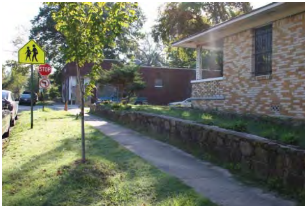
Figure 2-41. The brick house and mortared stone retaining wall at 1600 S. Park Street is depicted in photographs from 1957. Source: John Milner Associates, Inc., 2007.
