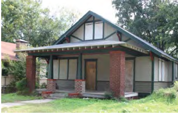
Figure 2-152. Brick porch columns. Source: John Milner Associates, Inc., 2007.
