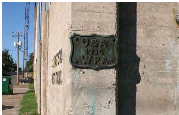
Figure 2-90. The 1936 WPA plaque mounted on the southwest corner of the wall surrounding Quigley Stadium. Source: John Milner Associates, Inc., 2007.
