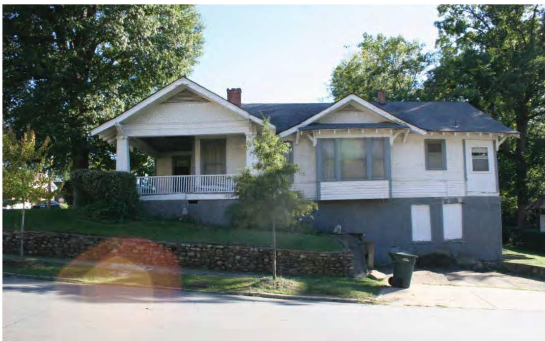
Figure 2-184b. The house and stone retaining wall at 1600 Dennison Street in 2007. Source: JMA, 2007.
