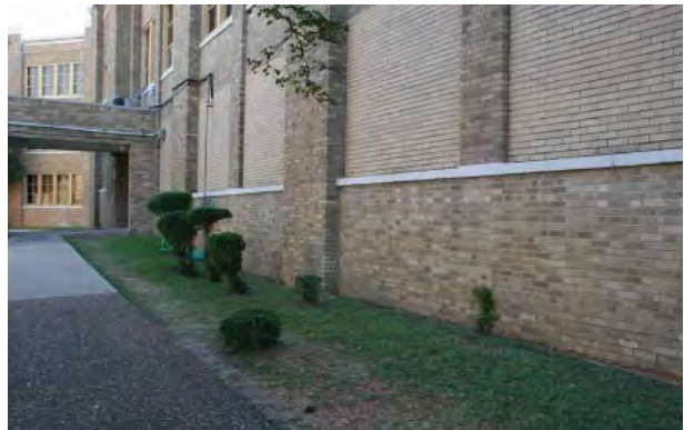
Figure 2-95. A covered walkway between the main school and the library. Source: John Milner Associates, Inc., 2007.
