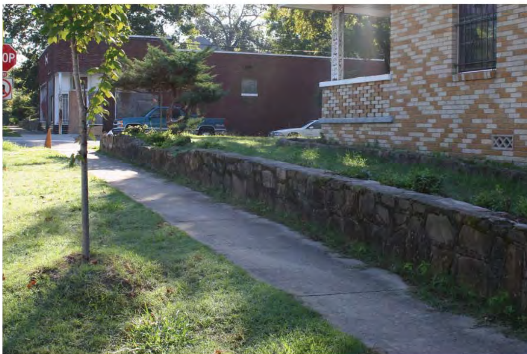
Figure 2-180b. Today, the house and stone wall appear to be in very much the same condition as they were in 1957-58. Source: John Milner Associates, Inc., 2007.
