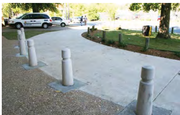
Figure 2-61. Concrete bollards, installed in 2007, at the east end entrance door. Source: John Milner Associates, Inc., 2007.
