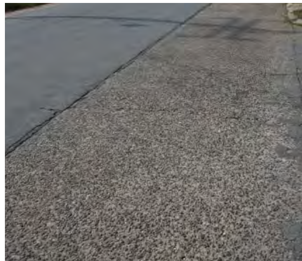
Figure 2-163. A broad exposed aggregate gutter or parking strip lines may of the streets. Source: John Milner Associates, Inc., 2007.
