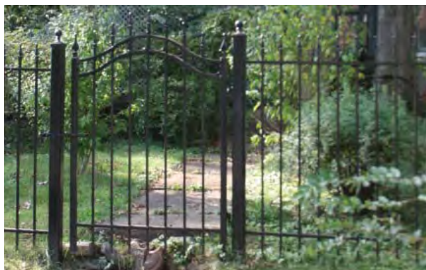
Figure 2-168. Metal fencing. Source: John Milner Associates, Inc., 2007.
