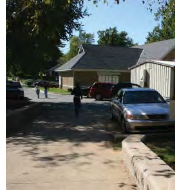
Figure 2-119. Views towards the neighborhood are also obstructed by the modular structures. Source: John Milner Associates, Inc., 2007.
