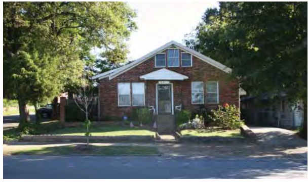
Figure 2-106. Post-war-era house at Rice Street and W. Sixteenth St. Source: John Milner Associates, Inc., 2007.
