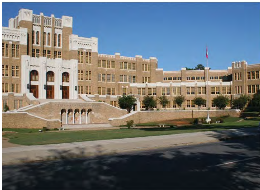
Figure 2-175b. In this recent view of the high school, many features are extant from the historic period. Missing, however, are the utility poles that once lined the west side of S. Park Street. Source: John Milner Associates, Inc., 2007.
