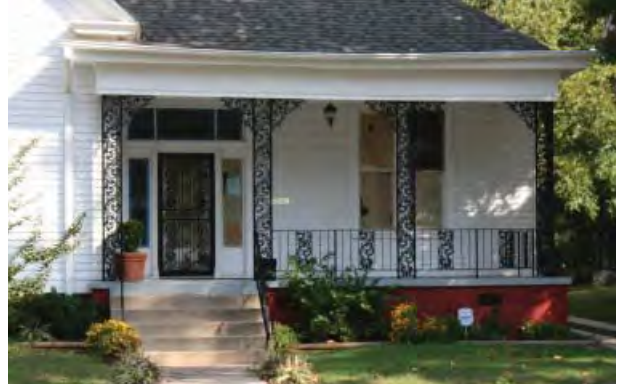
Figure 2-153. Ornamental metal porch columns. Source: John Milner Associates, Inc., 2007.
