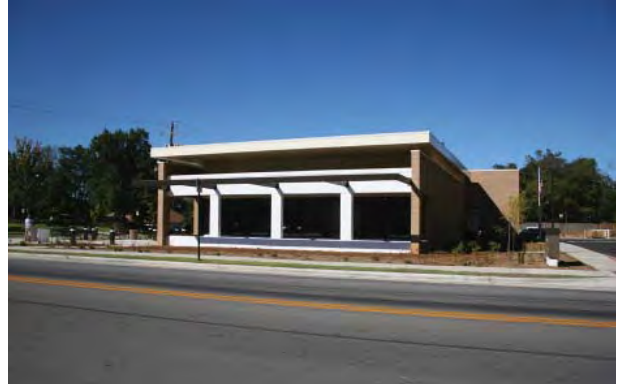
Figure 2-70. The south end of the NHS Visitor Center features glass windows, so that a view of the school forms the backdrop of its interior interpretive exhibits. Source: John Milner Associates, Inc., 2007.
