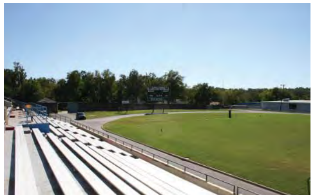
Figure 2-116. View of the surrounding wall from within the stadium. Source: John Milner Associates, Inc., 2007.
