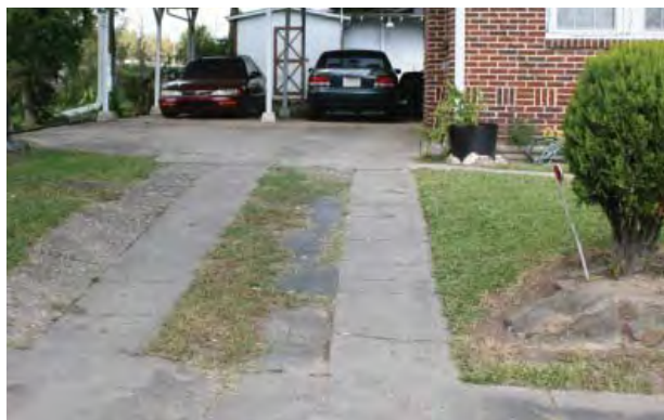
Figure 2-164. Residential driveways are frequently concrete two-tracks with a turf center. Source: John Milner Associates, Inc., 2007.
