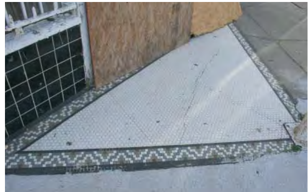
Figure 2-51. Ornamental ceramic tile at the threshold of the Capel Building (formerly Ponder's Drug Store). Source: John Milner Associates, Inc., 2007.
