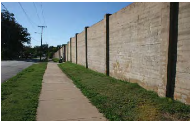
Figure 2-115. The poured concrete wall that surrounds Quigley Stadium. Source: John Milner Associates, Inc., 2007.
