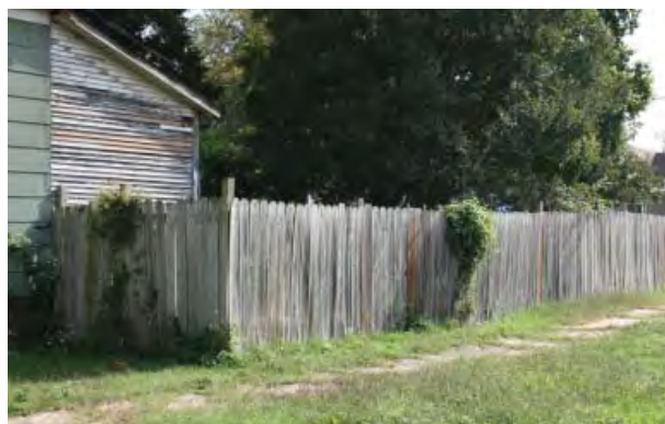
Figure 2-173. Wood board privacy fence. Source: John Milner Associates, Inc., 2007.
