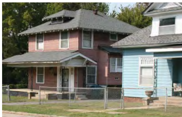
Figure 2-171. Chain link fencing. Source: John Milner Associates, Inc., 2007.
