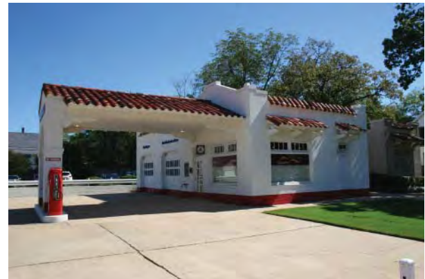
Figure 2-42. The Magnolia Mobil service station, where journalists phoned in their stories in 1957, was rehabilitated to its ca. 1950s appearance in 1997. Source: John Milner Associates, Inc., 2007.
