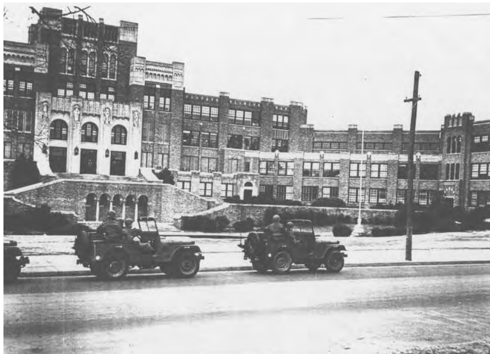
Figure 2-175a. This photograph from ca. 1957-58 shows the utility pole and overhead utility lines that defined the space of S. Park Street on its west side. Source: Central High Museum, Inc., COLL.B.12.I.257, no date, National Park Service, Little Rock Central High School National Historic Site.
