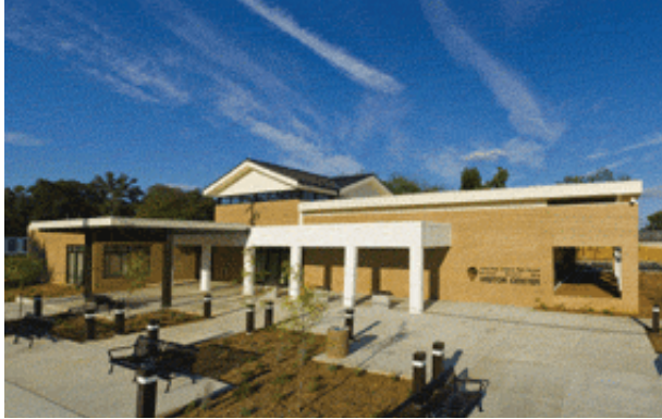
Figure 2-69. The Little Rock Central High School NHS Visitor Center opened in the fall of 2007. Source: John Milner Associates, Inc., 2007.
