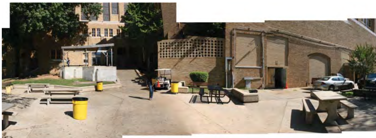
Figure 2-87. This panoramic photomontage illustrates the complex rear facade of the high school building and the variety of uses hosted there. Access to the lower level is through the garage doors to the right. Source: John Milner Associates, Inc., 2007.
