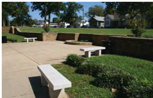
Figure 2-58. Ten concrete commemorative benches in the sunken plaza area are inscribed with the names of the “Little Rock Nine;” the tenth represents all past, present, and future students of the school. Source: John Milner Associates, Inc., 2007.
