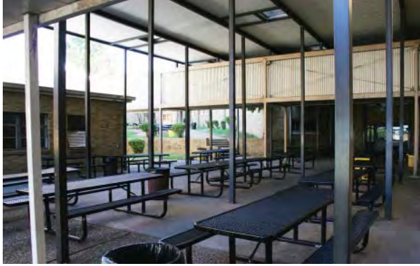
Figure 2-92. A modern overhead structure on the west side of the school. Source: John Milner Associates, Inc., 2007.
