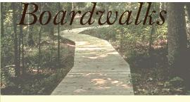
Boardwalk installation involves construction techniques dependent on the material chosen, and their width and length. All boardwalks need curbing, but where 30" or more above grade should also have a handrail.
